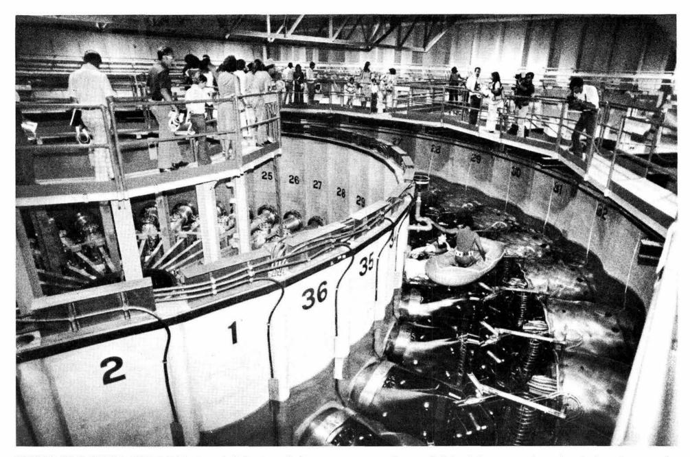
PARTICLE BEAM FUSION ACCELERATOR—Formal dedication of this new facility, designed for pulsed power experiments leading to the demonstration of inertially confined fusion, took place last Saturday, Aug. 2. Some of the
